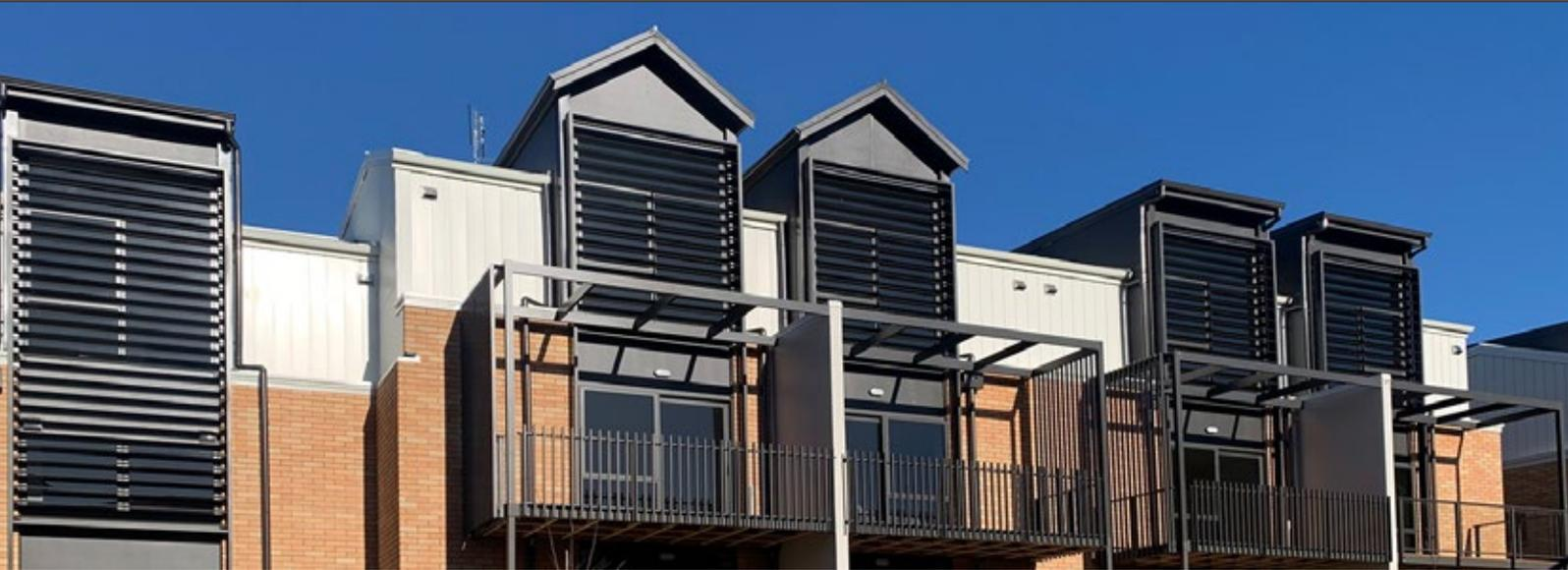
Aluminium louvres are a great solution to urban design requirements. They can be used to provide privacy, protection from the elements, or integrated into balustrade systems to form part of your safety from falling solution. Spectrum have a range of systems to meet your needs. Contact our team for individual products details.
